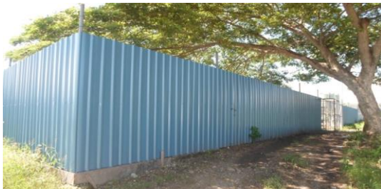
Figure 5. The Newly Fenced Timber yard
